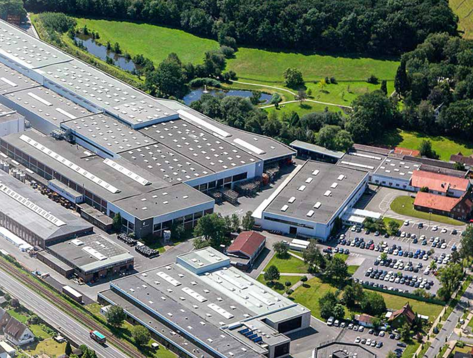
Headquarters of the Craemer Group in Herzebrock-Clarholz, Germany
